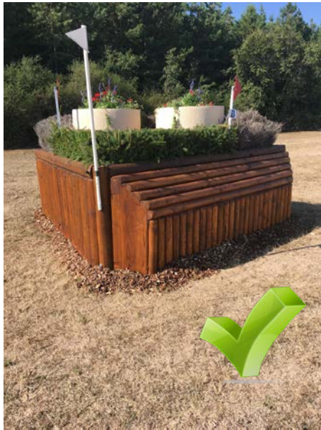
Good example of a sloped leading edges with the bottom filled.
