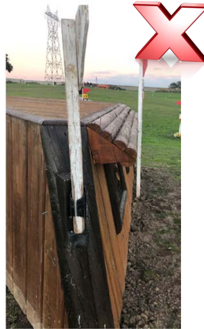
Bad example of fence: the front of the leading edge may well be sloped at 45 degrees but it is "false" leading edge, with no filling under with the risk that a horse can catch its leg or boot on its way up
